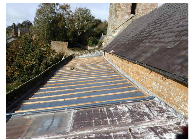
SOUTH AISLE ROOF
