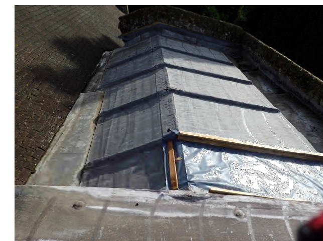
ORGAN CHAMBER ROOF
